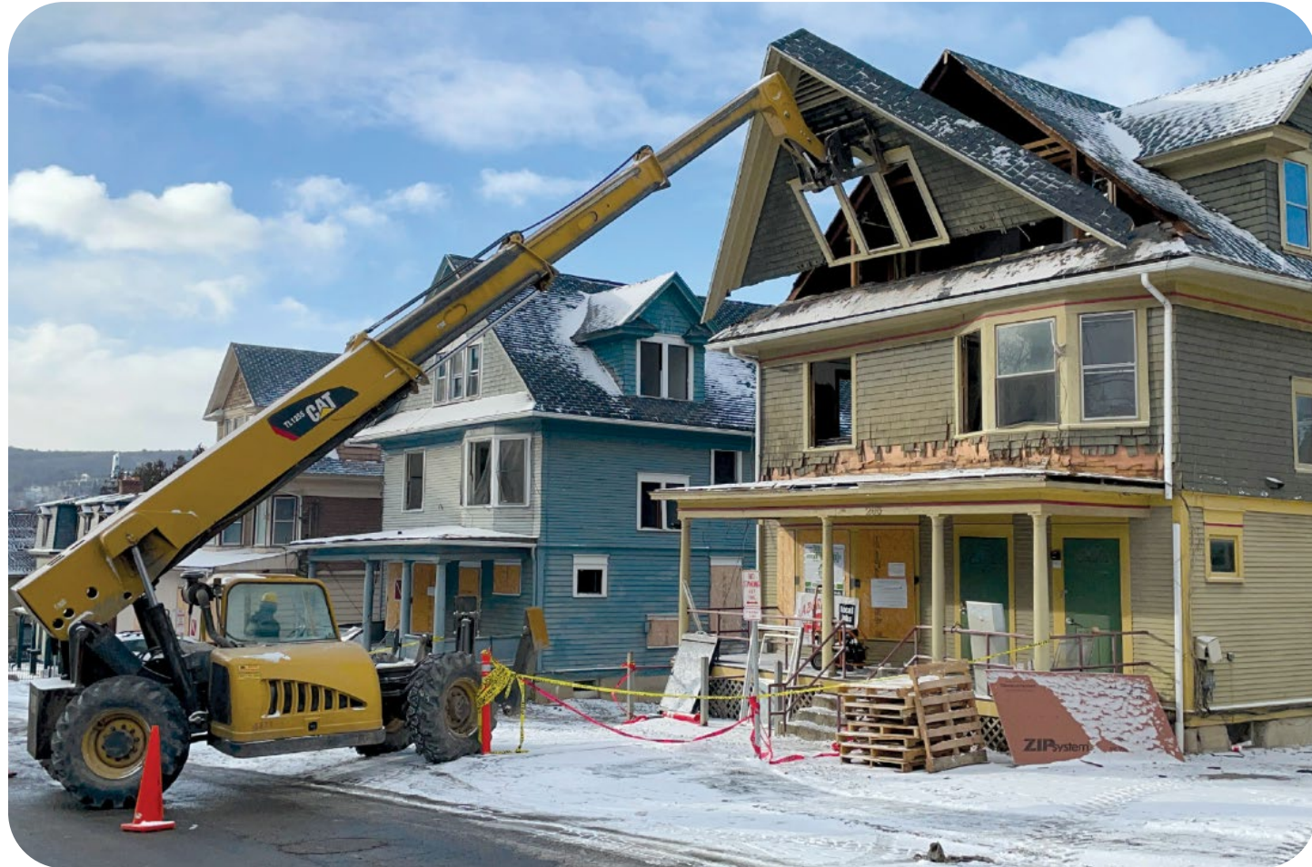
Deconstruction in progress, courtesy of Felix Heisel
