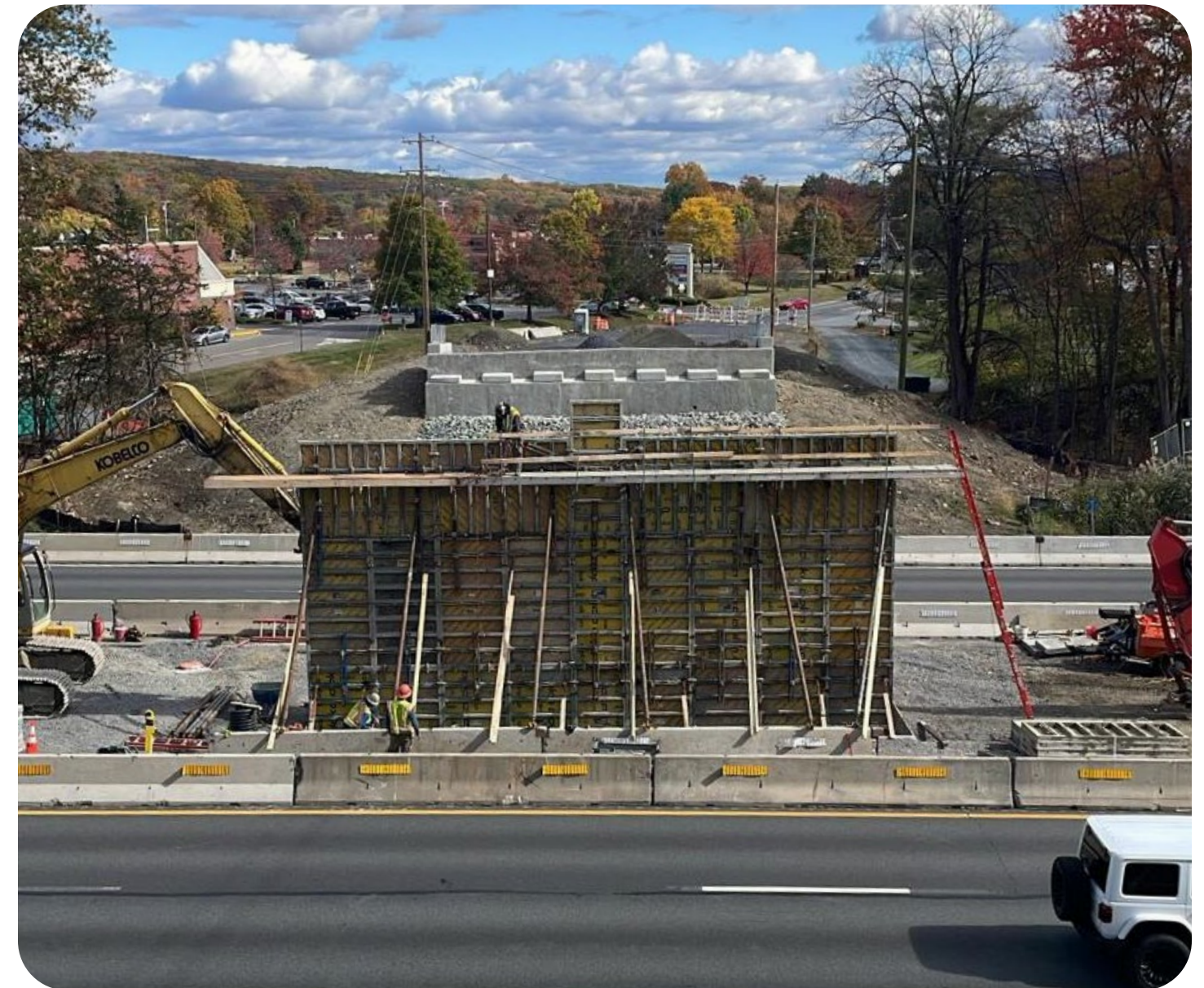
NYSDOT deployment of concrete with Pozzotive® ground-glass pozzolan, Courtesy of Bryan Concrete and Supply
