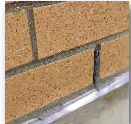
90% Open mesh "Weep Vents" Compression fit
