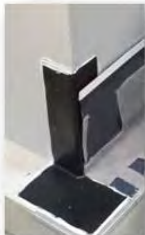
Prefab corners & end dams
