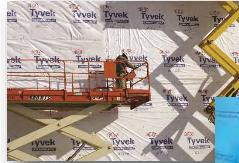
Mechanically Attached Sheet
