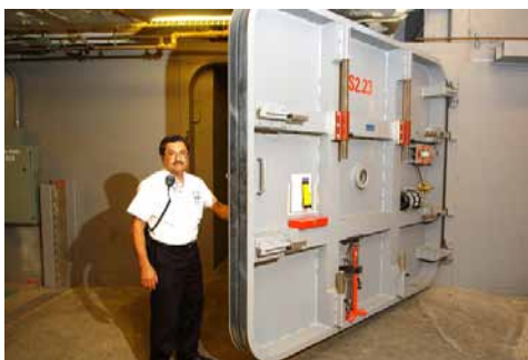
Watertight submarine door for creation of a protected infrastructure space. Photo credit: FEMA
