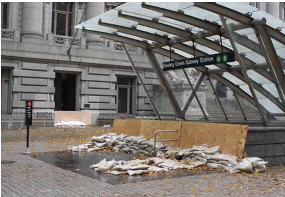
Temporary flood barriers were constructed prior to the storm at vulnerable entrances. Photo credit: Flickr / MTA Photos Photostream
