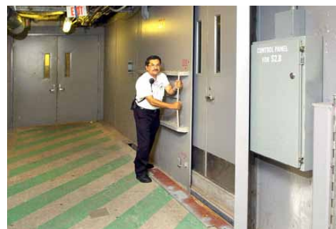
Watertight submarine door for protection of critical equipment within an unprotected passageway. Photo credit: FEMA
